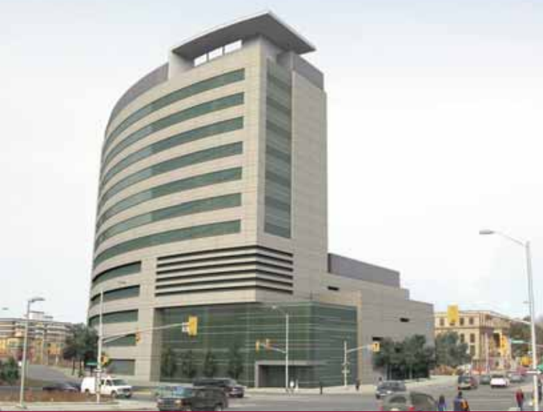
University of Ottawa Desmarais Building and new home of the School of Management. Estimated occupancy date, fall 2007.
